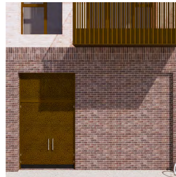
Figure 6.93: Perforated metal panels in refuse doors
