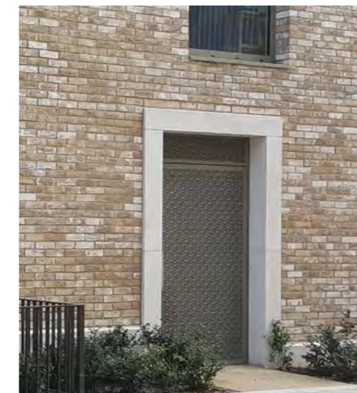
Figure 6.94: Precedent: perforated metalwork
