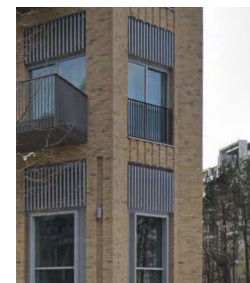
Figure 6.98: Precedent: use of vertical metal bars
