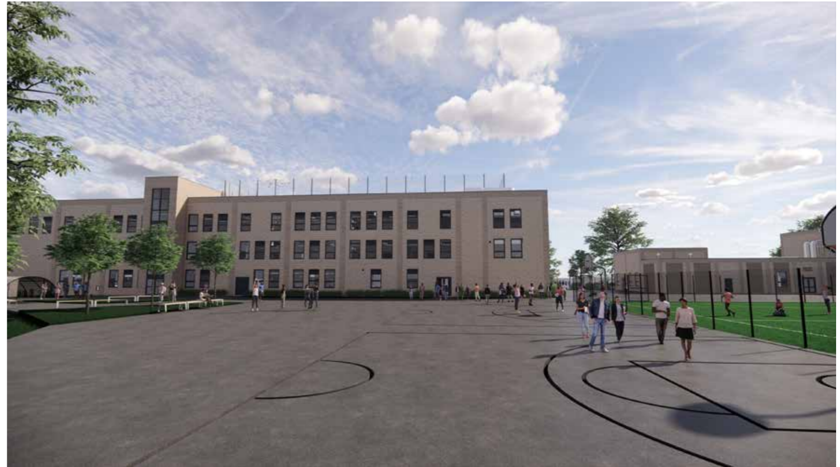
Exterior View of the School from the key Northeast corner
