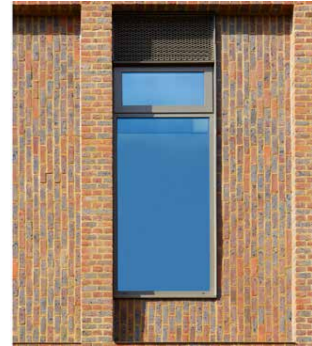
Examples of brick bonding and expressed structure
