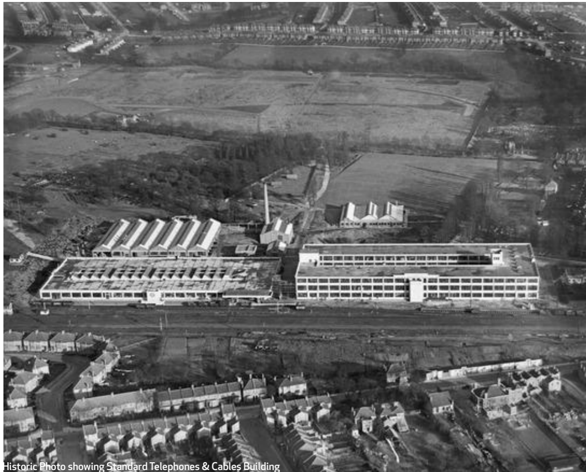
Historic Photo showing Standard Telephones & Cables Building
