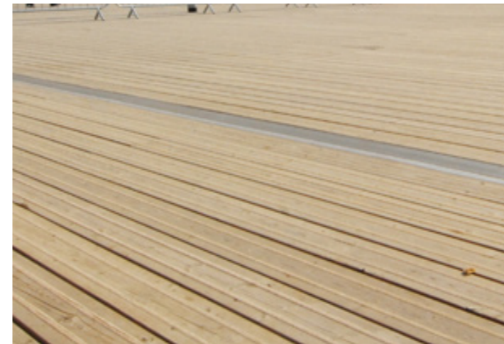
Timber decking Timber walkway in open space
