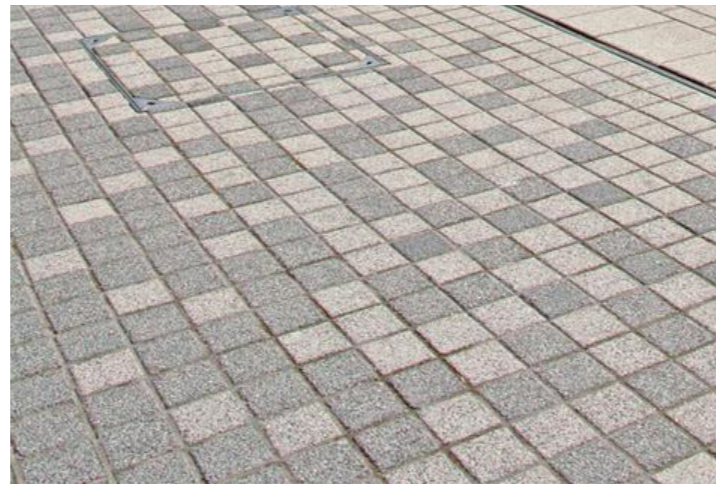
Type 2 Pedestrian cross: concrete conservation paving block 100 x 100 x 80 mm - Sliver grey
