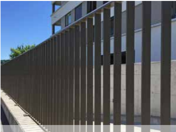
Pedestrian guardrail railings
