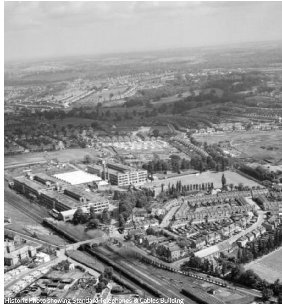
Historic Photo showing Standard Telephones & Cables Building
