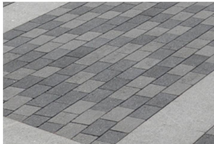
Type 3 - Pedestrian path: concrete conservation paving block 200 x 400 x 80 mm - Mixture of 2 tone of grey
