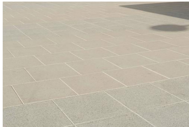
Type 4 - Pedestrian path: concrete conservation paving block 400 x 400 x 50 mm - Sliver grey
