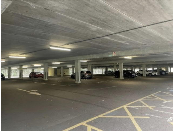
Figure 2-45 Multi-Storey Car Park, Ground Level
