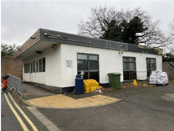
Figure 2-43 Unidentified Ancillary Structure (Northern Façade)
