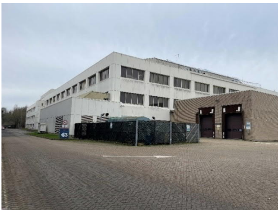
Figure 2-26 Building 4 (Southern Façade)
