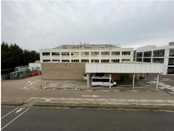
Figure 2-27 Building 4 (South-Eastern Façade)
