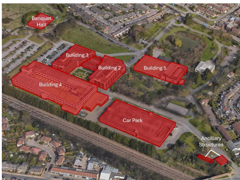
Figure 4-1 Structures Due for Demolition
