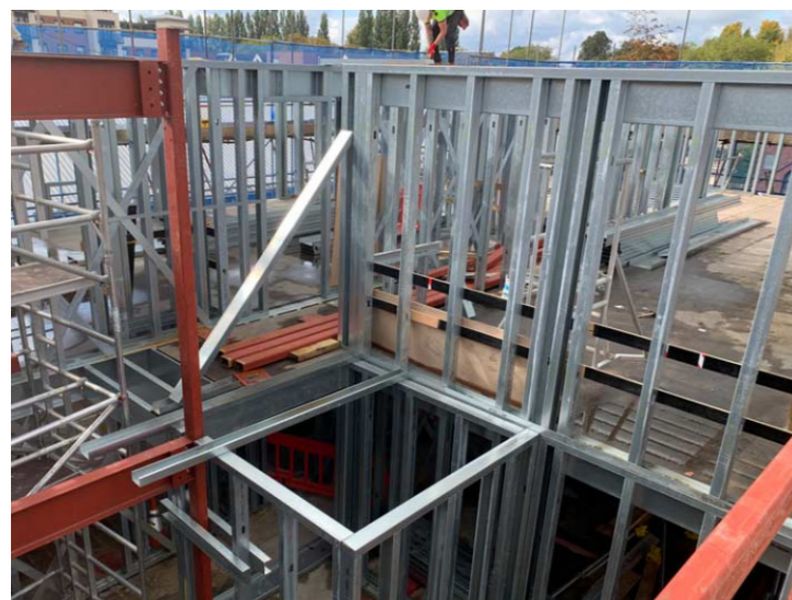
04 Steel Structure/ Metsec outer Wall
