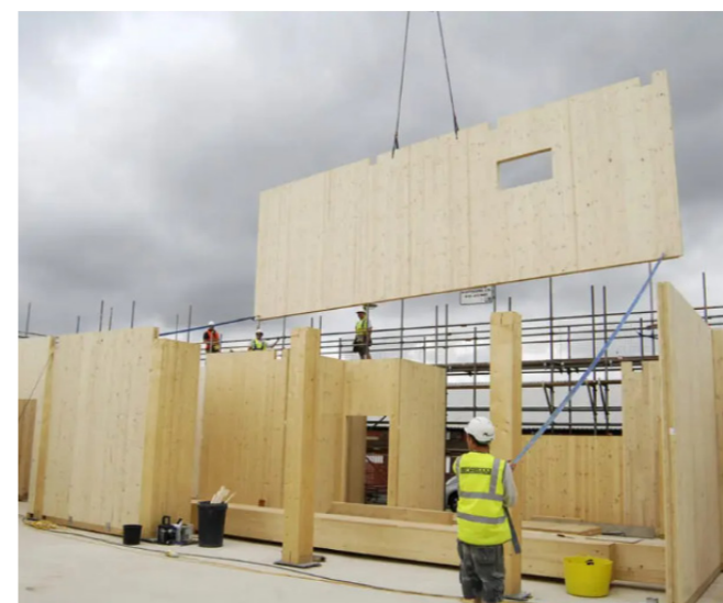
06 Cross Laminated Timber (CLT) Walls & Floors
