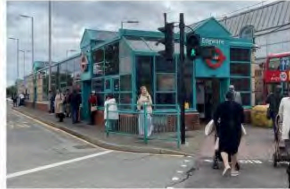
covered bus station with 5 stands
