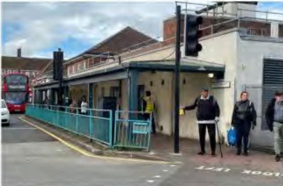
Covered walk from tube station to
