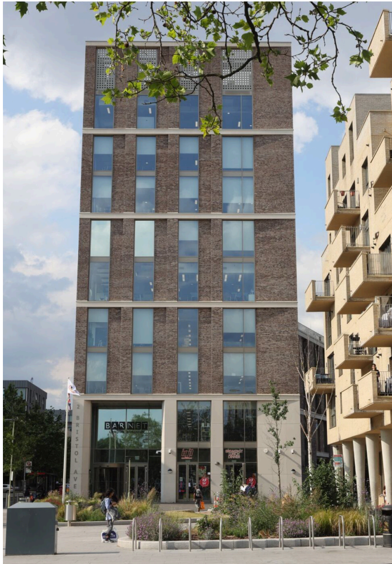
Collindale Offices, HawkinsBrown © Barnet Council
