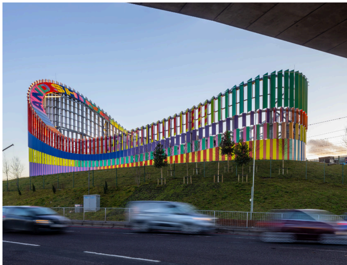
Brent Cross Town Substation by IF_DO © Jason Hawkes
