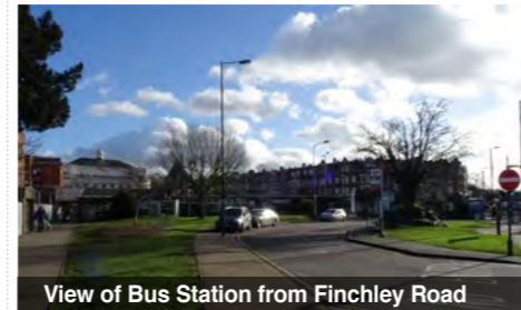
View of Bus Station from Finchley Road
