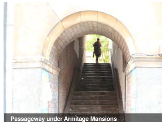
Passageway under Armitage Mansions
