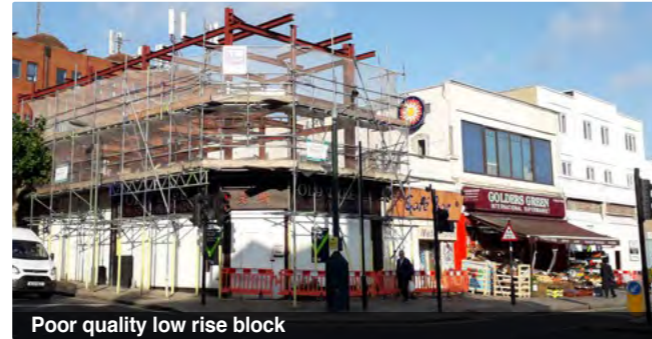
Poor quality low rise block
