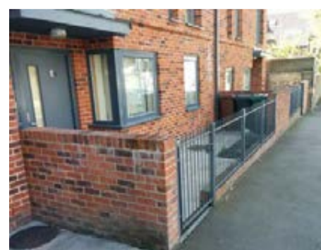
Semi-concealed bin store in private gardens Hammond Court, Waltham Forrest
