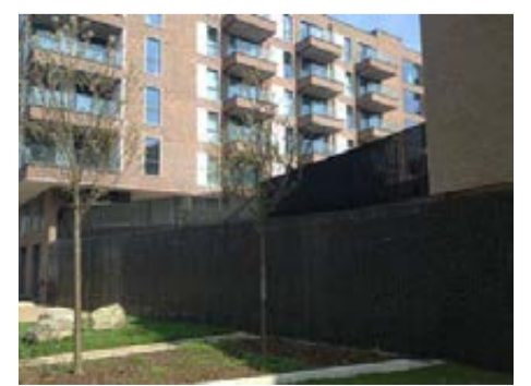
Podium parking concealed behind textured metalwork, Thames Barrier East
