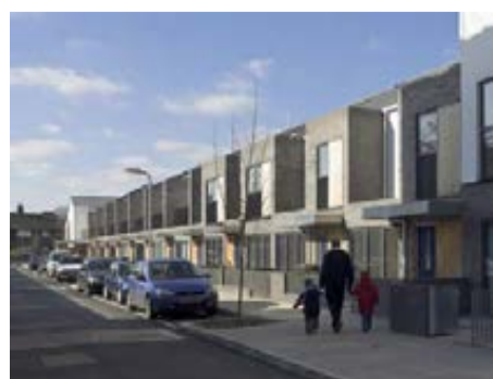
Dark brick finishes, Queensbridge Quarter, Levitt Bernstein
