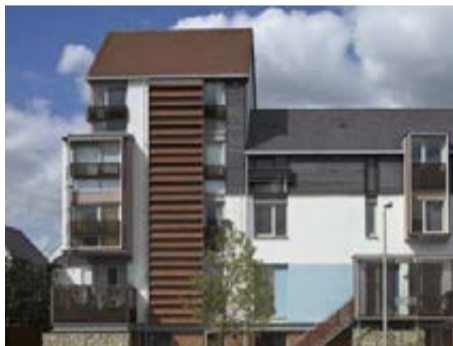
Height and change in material to corner Abode, Newhall
