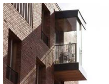
Articulation of the elevational line, Timberyard, Dublin
