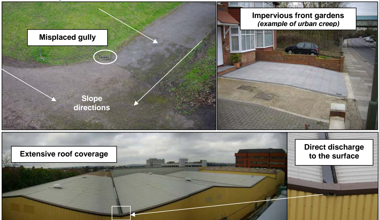
Figure B5 - Examples of drainage arrangements and building standards to avoid during re-development
