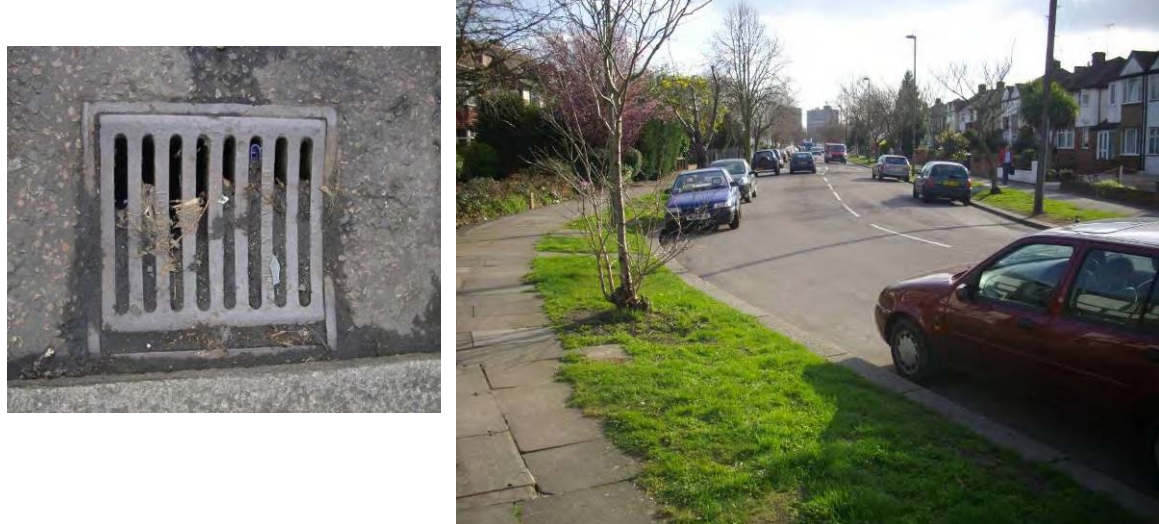
Figure B4 - Example of localised drainage issues: blocked gully at Colindeep Lane and low point at Rushgrove Avenue
