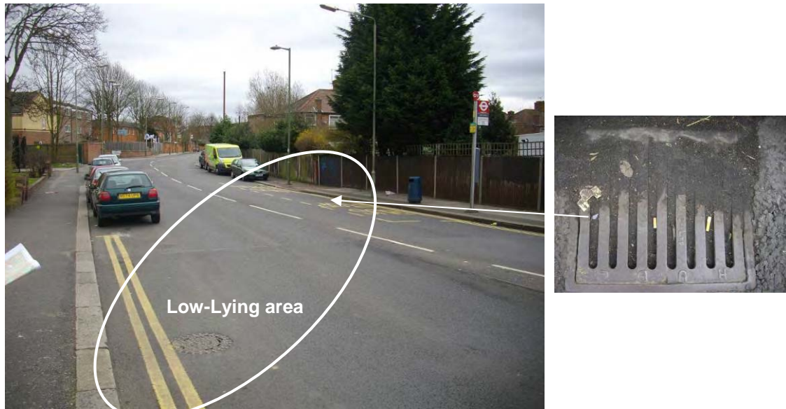
Figure B4 - Example of localised drainage issues: blocked gully at Colindeep Lane and low point at Rushgrove Avenue
