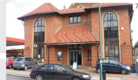
Renovation to Church with predominant use of brick
