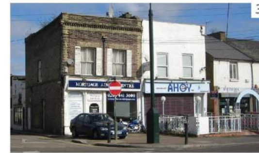
Poor quality buildings at East Barnet Road/Victoria Road junction
