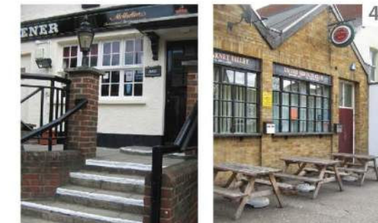
Small-scale buildings along East Barnet Road add architectural character to High Street
