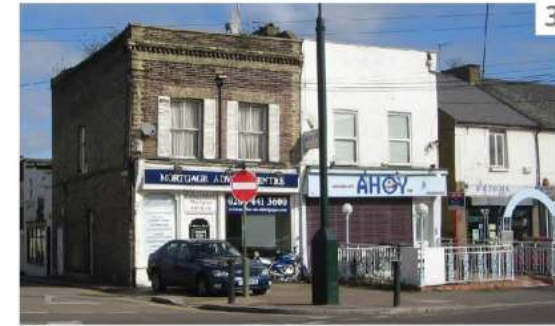
3 Poor quality buildings at East Barnet Road/Victoria Road junction
