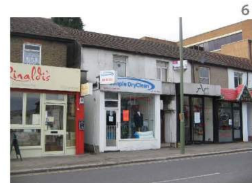
6 Low quality buildings along East Barnet Road
