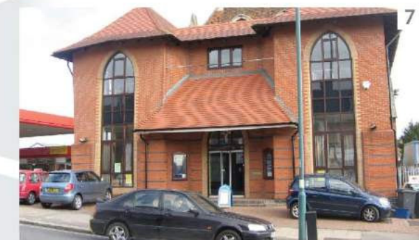
7 Renovation to Church with predominant use of brick
