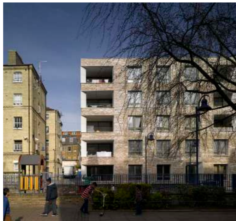
Terraces contained and integrated into the wider facade
