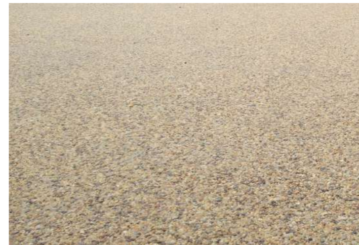
Resin bound gravel Pedestrian path in open space
