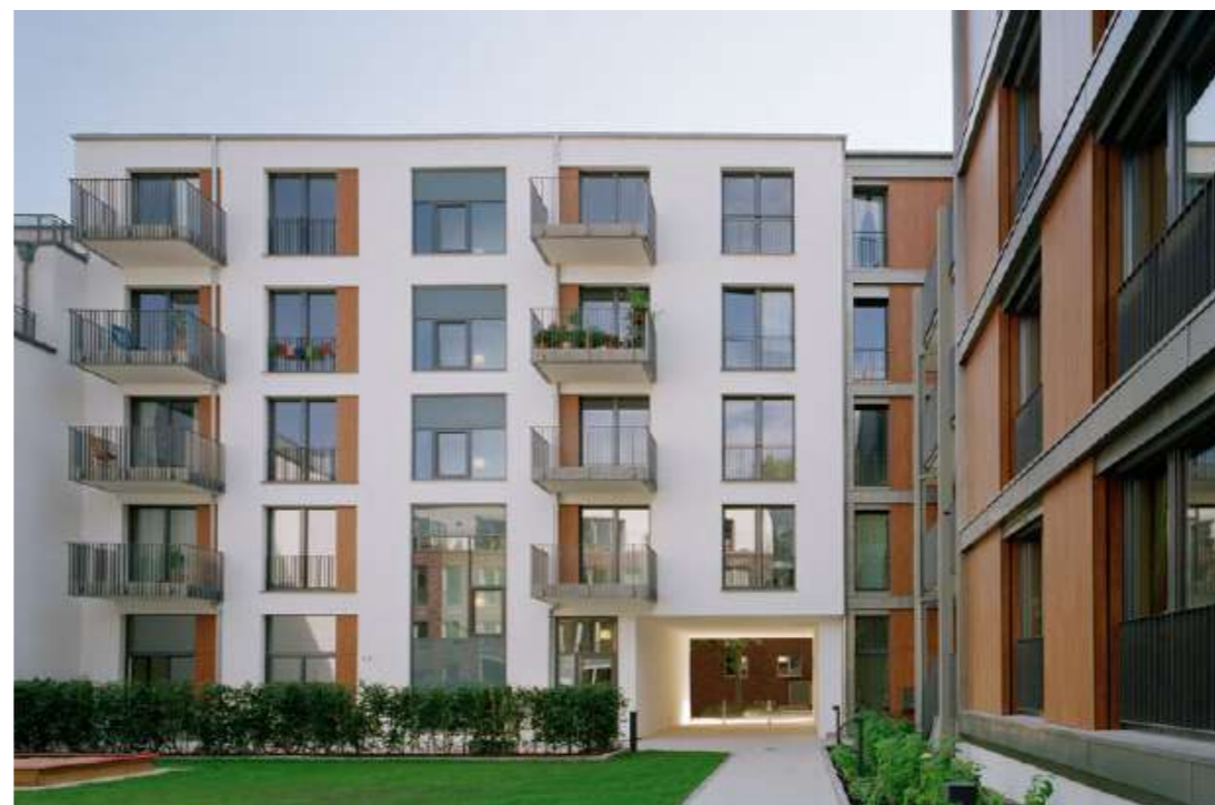
Courtyards provided with light-reflecting finishes
