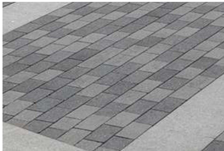
Pedestrian path: concrete conservation paving block 200 x 400 x 80 mm - Mixture of 2 tone of grey
