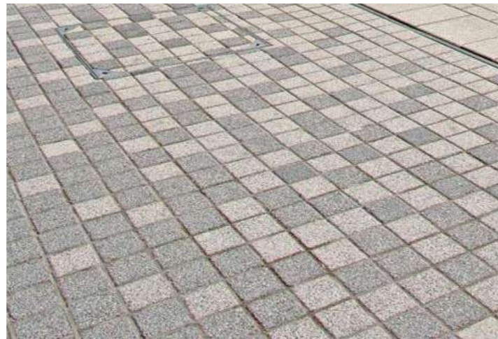
Pedestrian crossings/raised tables: concrete conservation paving block 100 x 100 x 80 mm - Sliver grey
