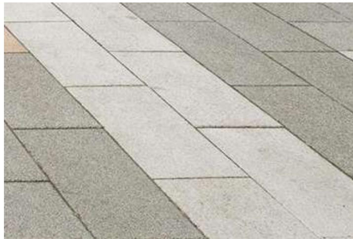
Public realm: concrete conservation paving block 300 x 600 x 80 mm - Mixture of 2 tone of grey
