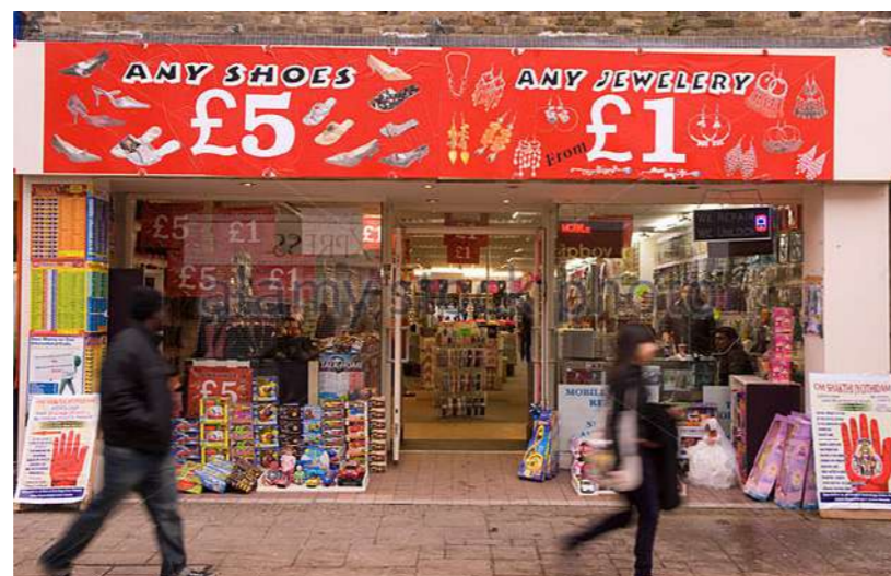
Poorly managed, poorly designed, poorly proportioned ground level uses within facade
