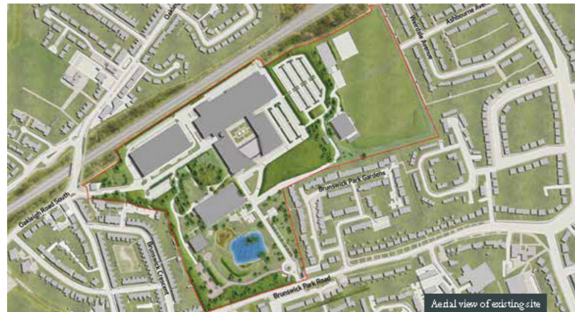
Aerial view of existing site
