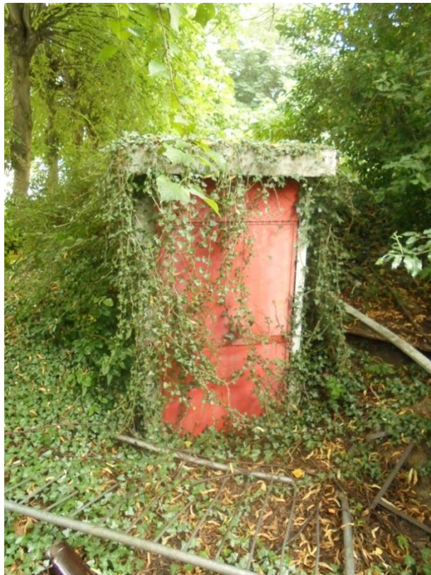
Plate 9.8 Northwest-facing view of entrance to former STC air raid shelters (Site 62)
