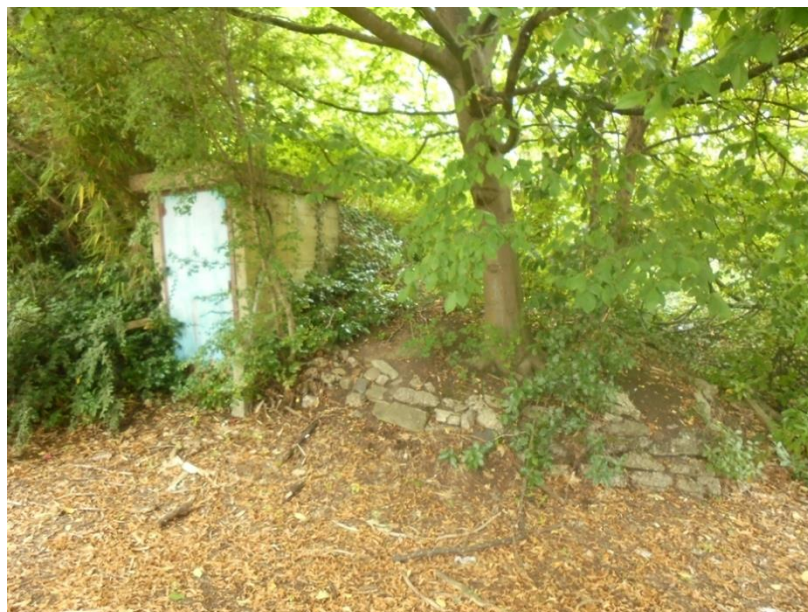
Plate 9.6 Northwest-facing view of entrance to former STC air raid shelters (Site 62)
