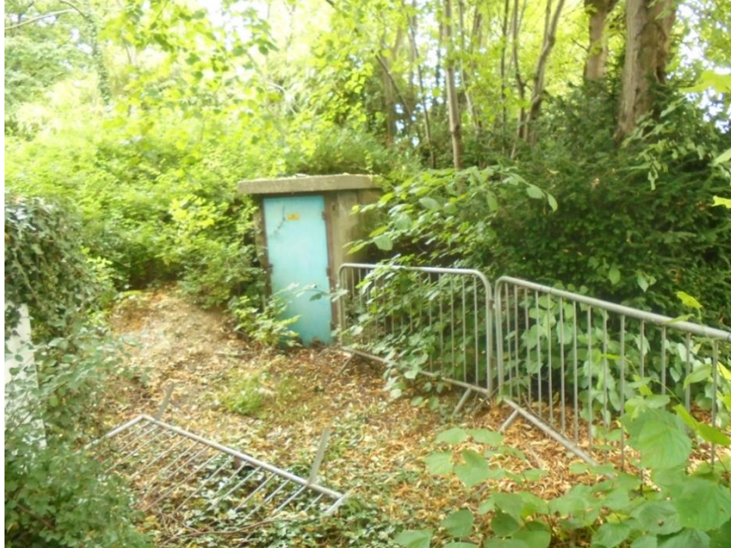
Plate 9.7 Southeast-facing view of entrance to former STC air raid shelters (Site 62)
