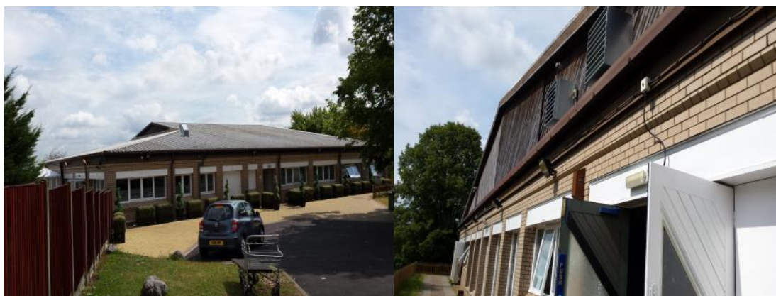
Photograph 11 & 12. Building B3 external features
