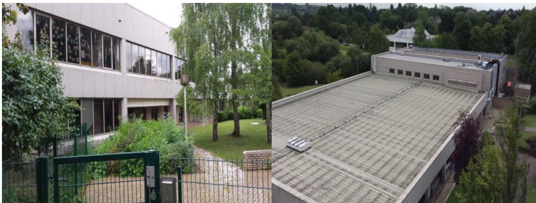
Photographs 16 & 17. Building B7 external and roof features (seen from B1a)
