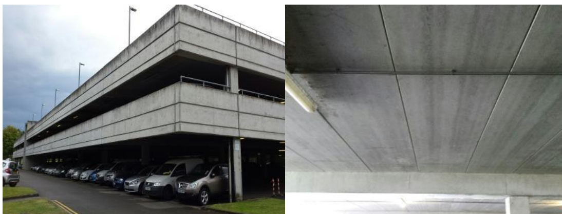
Photograph 20 & 21. Building B10 car park
