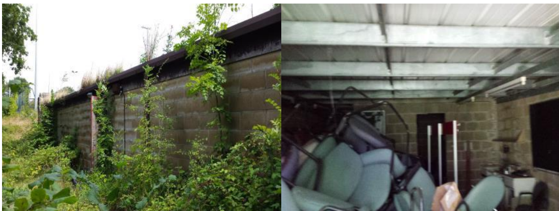
Photographs 9 & 10. Showing the external and internal features of building B2
