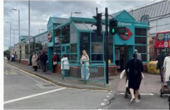
covered bus station with 5 stands
